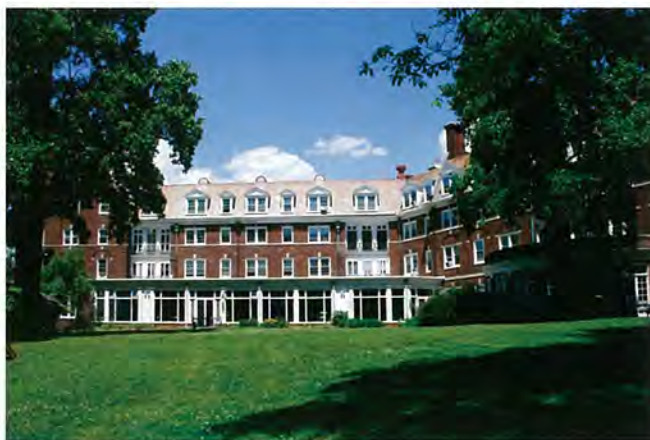
Photo: Courtesy of PZS Architects LLC Cross Properties is renovating the Palmer Seminary into apartments.
